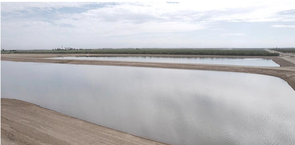
Basin #11 actively recharging
