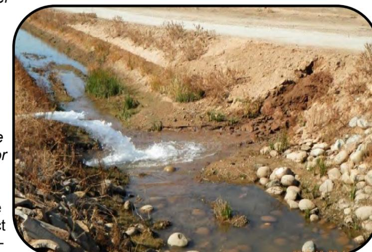
Above: Canal bank erosion from illegal pipeline discharge
